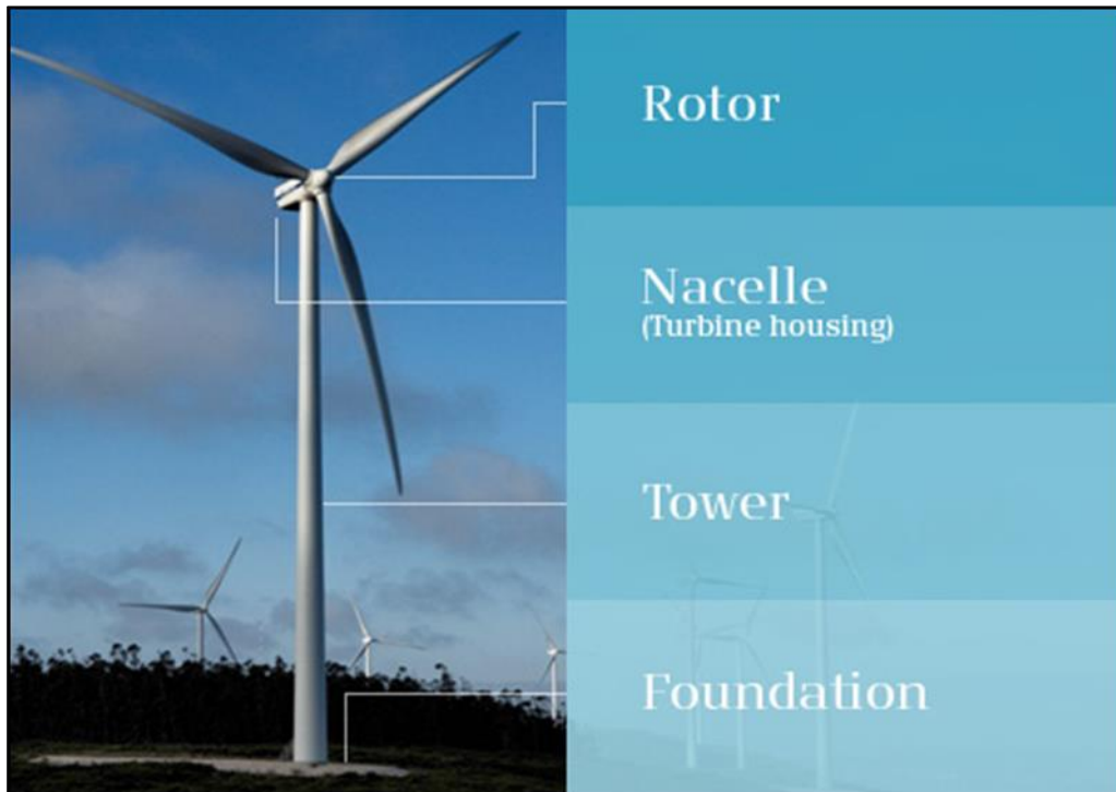
Plate 4-1 Wind turbine components
