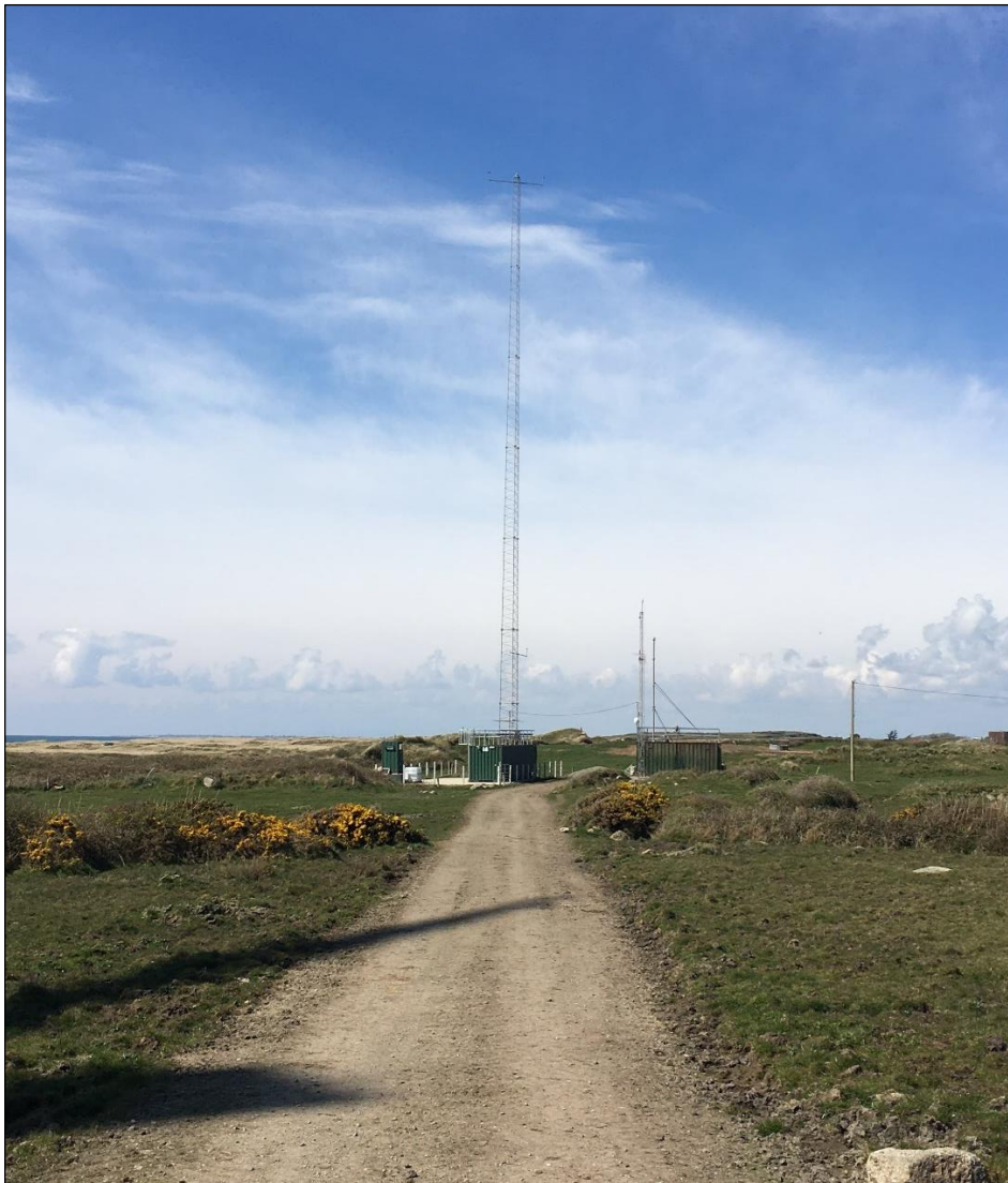
Plate 4-3 Existing meteorological mast and air monitoring mast
